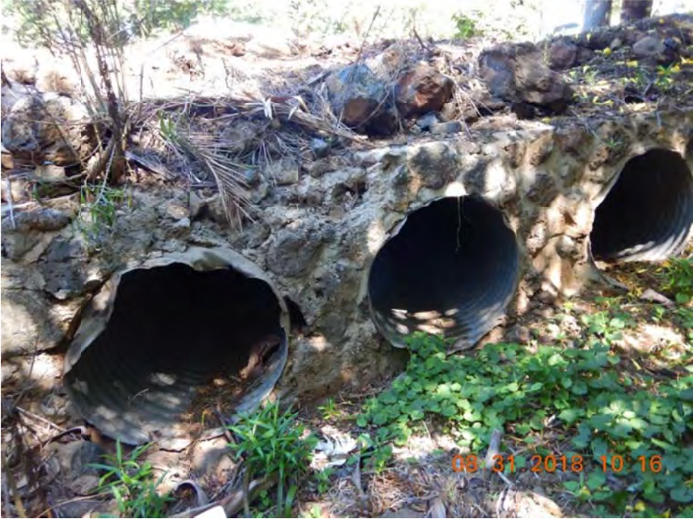
Photo 2: Stand on stream, look toward Culvert 26 inlet
