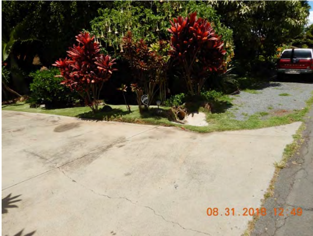
Photo 3: Look toward roadside culvert inlet at TMK: 2-1-019: 062
