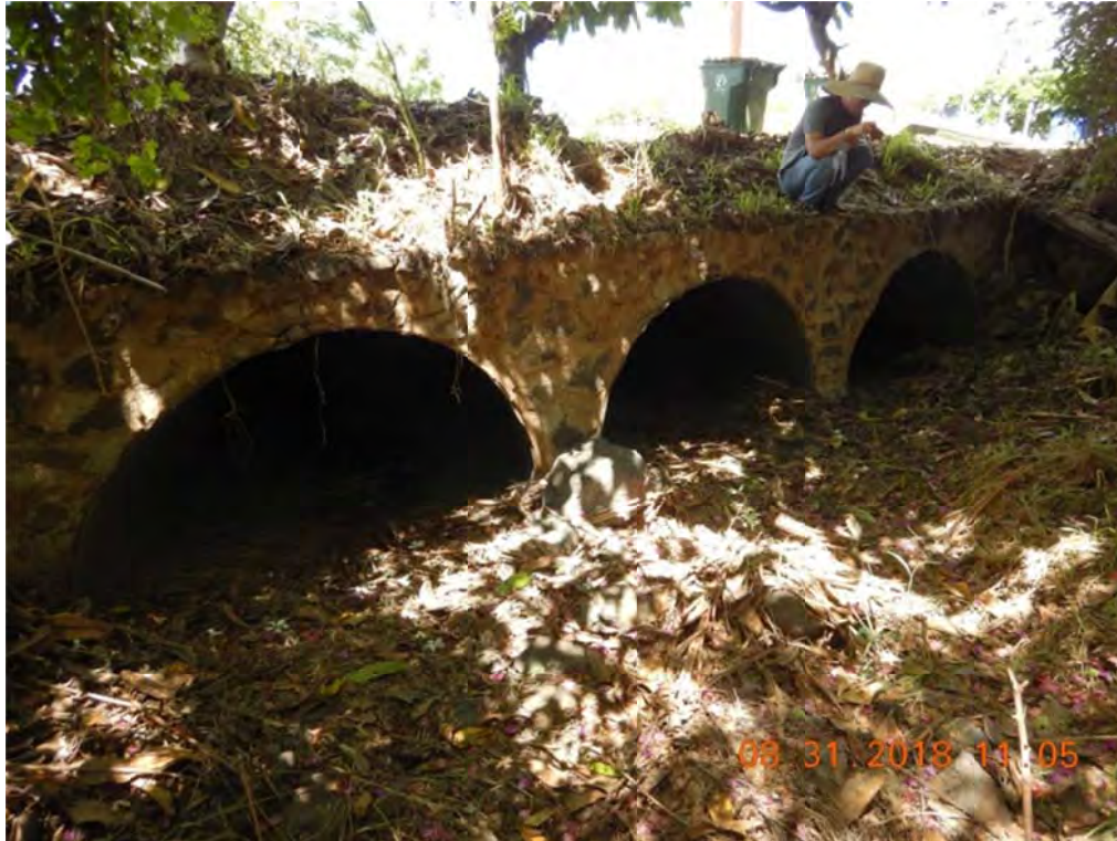
Photo 1: Stand on Stream, look toward Culvert 43 inlet
