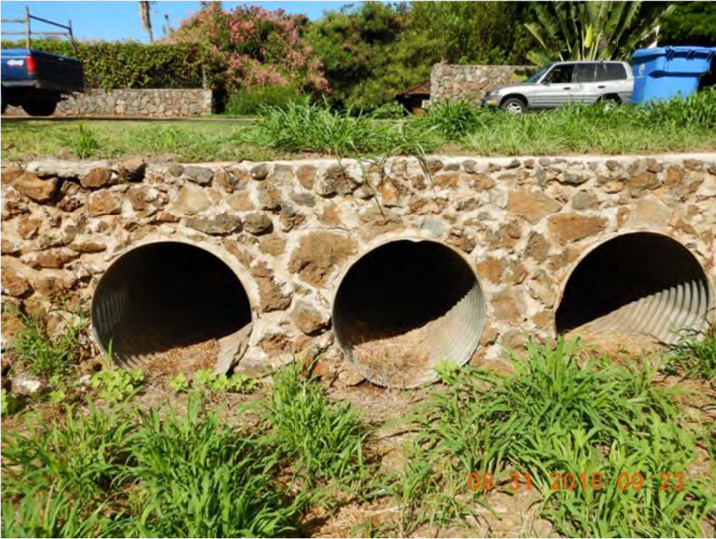
Photo 4: Close-up view of Culvert 32 inlets
