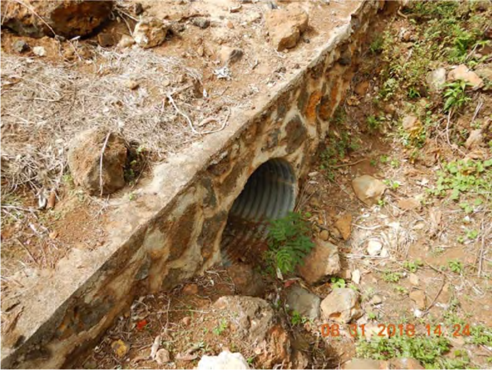
Photo 2: Stand on left bank, look toward Culvert 21 inlet
