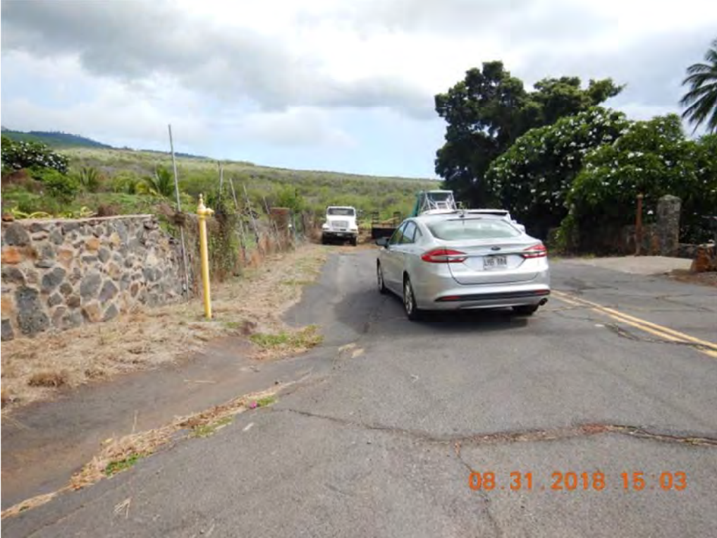
Photo 5: Kumulani Dr. roadside swale (south side) continues to Hoala Dr.
