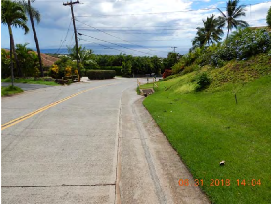
Photo 1: Stand on Kumulani Dr, look downstream toward Culvert 12 (Road side DI)
