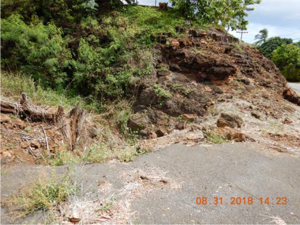
Photo 1: Stand on Hookipa Pl, look toward upstream of Culvert 21
