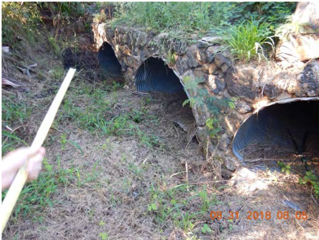
Photo 16: Stand on stream, look toward Culvert 36 inlet
