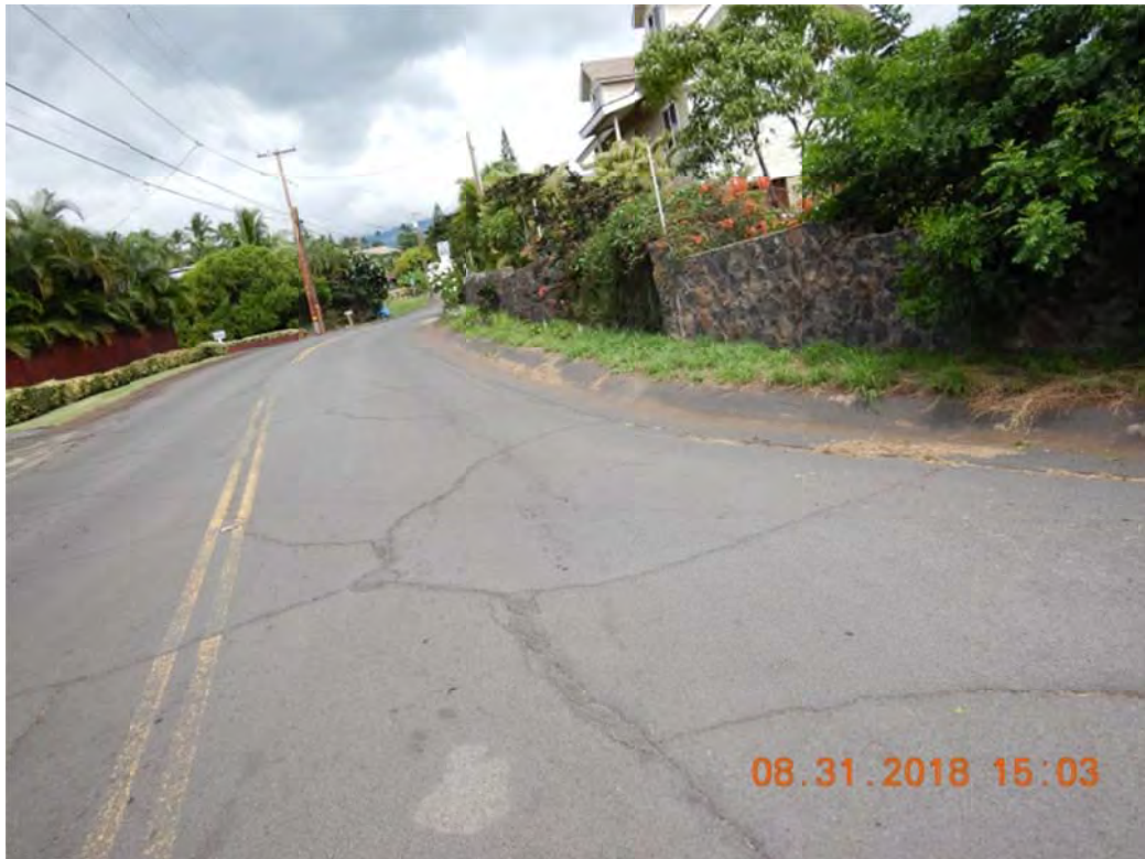
Photo 4: Kumulani Dr. roadside swale (south side)
