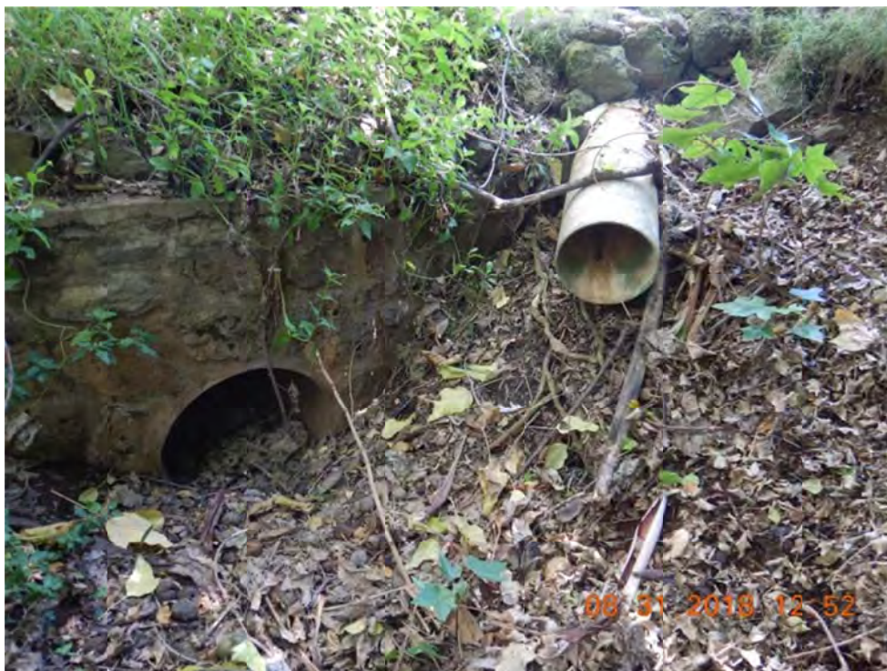
Photo 2: Downstream view of Culvert 8 and roadside culvert (12") outlets
