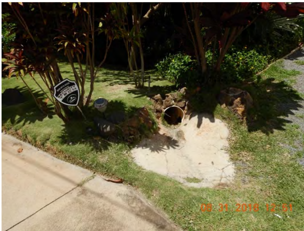
Photo 4: Close-up view of roadside culvert inlet at TMK: 2-1-019: 062
