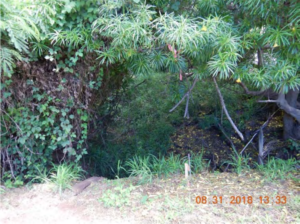
Photo 1: Stand on Kupulau Dr, look toward upstream of Culvert 7
