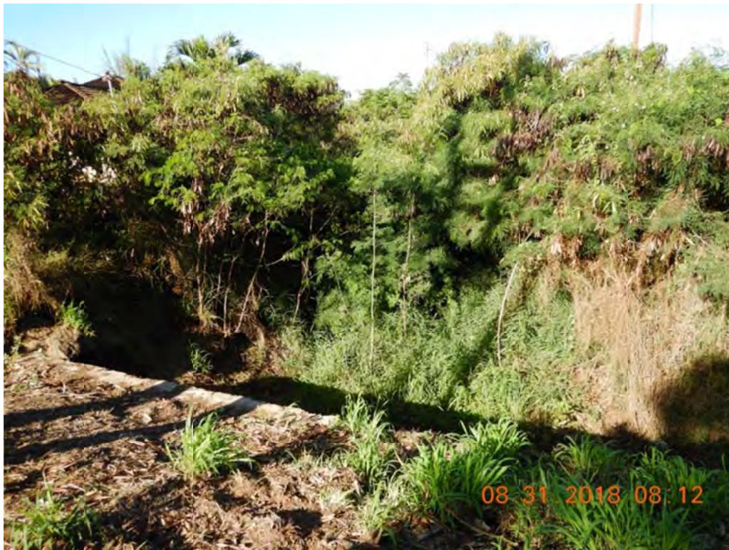
Photo 18: Stand on Akala Dr., look toward downstream channel of Culvert 36 outlet
