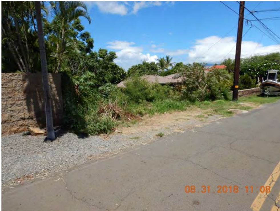
Photo 3: Stand on Kehala Dr, look downstream toward Culvert 43
