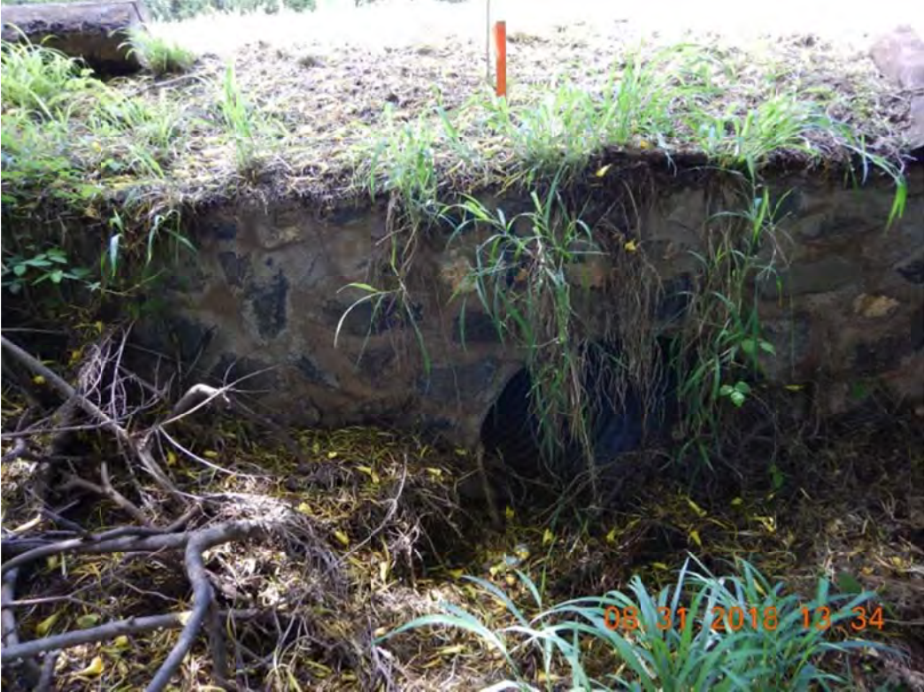
Photo 2: Stand on stream, look toward Culvert 7 inlet
