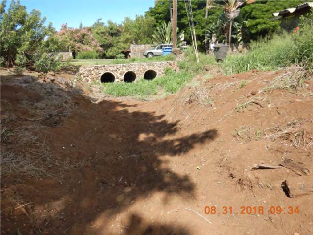
Photo 3: Stand on stream, look downstream toward Culvert 32 inlet
