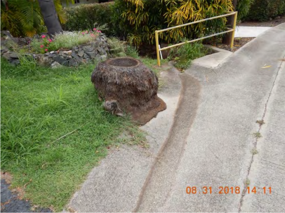
Photo 3: Existing DI across Culvert 12 at the opposite side of Kumulani Dr.
