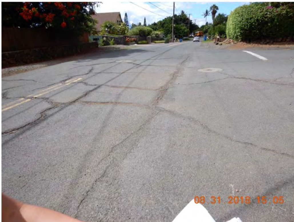
Photo 2: Stand on south side of the intersection, look toward the intersection
