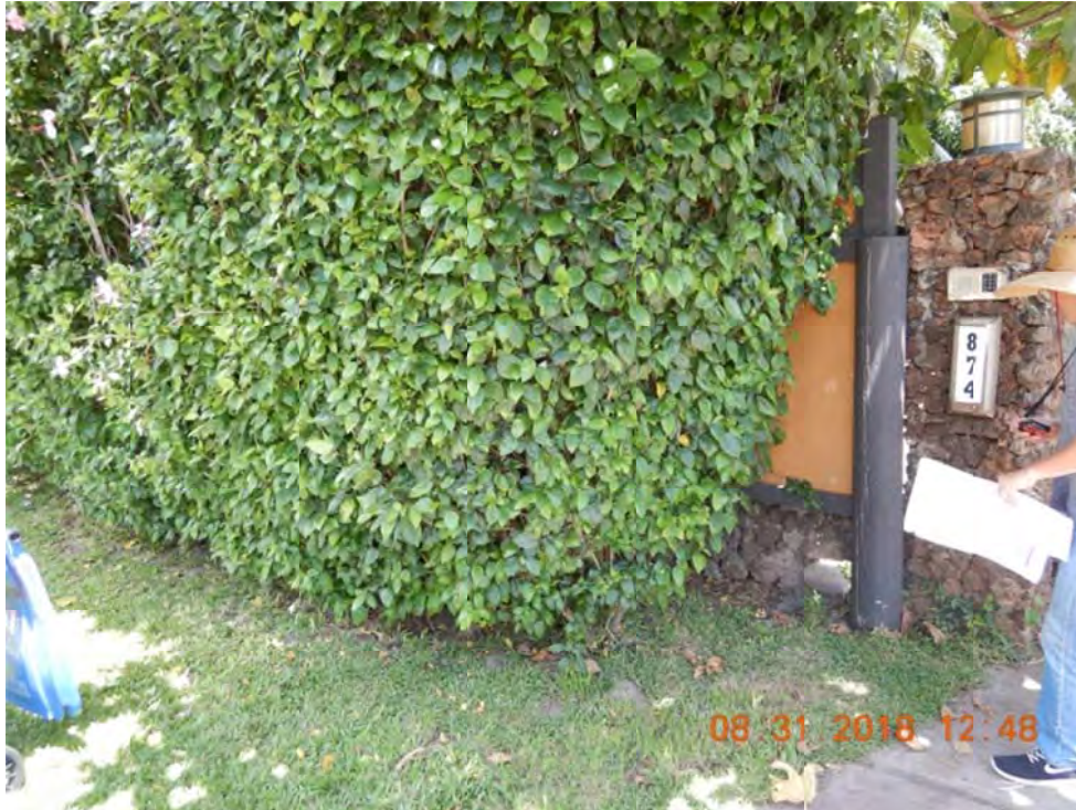
Photo 1: Upstream of Culvert 8 is not accessible (private property)
