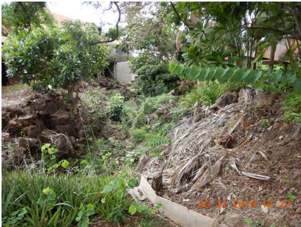
Photo 4: Stand on right bank, look toward downstream of Culvert 21
