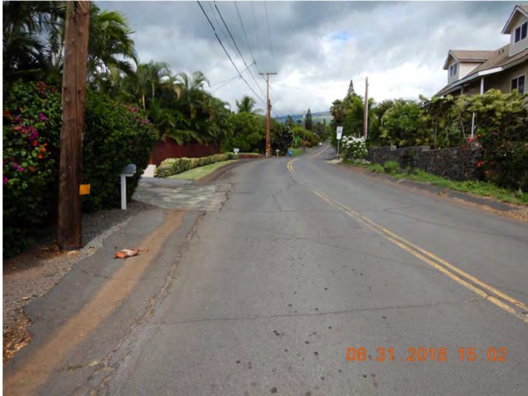
Photo 3: Kumulani Dr. roadside swale (north side)
