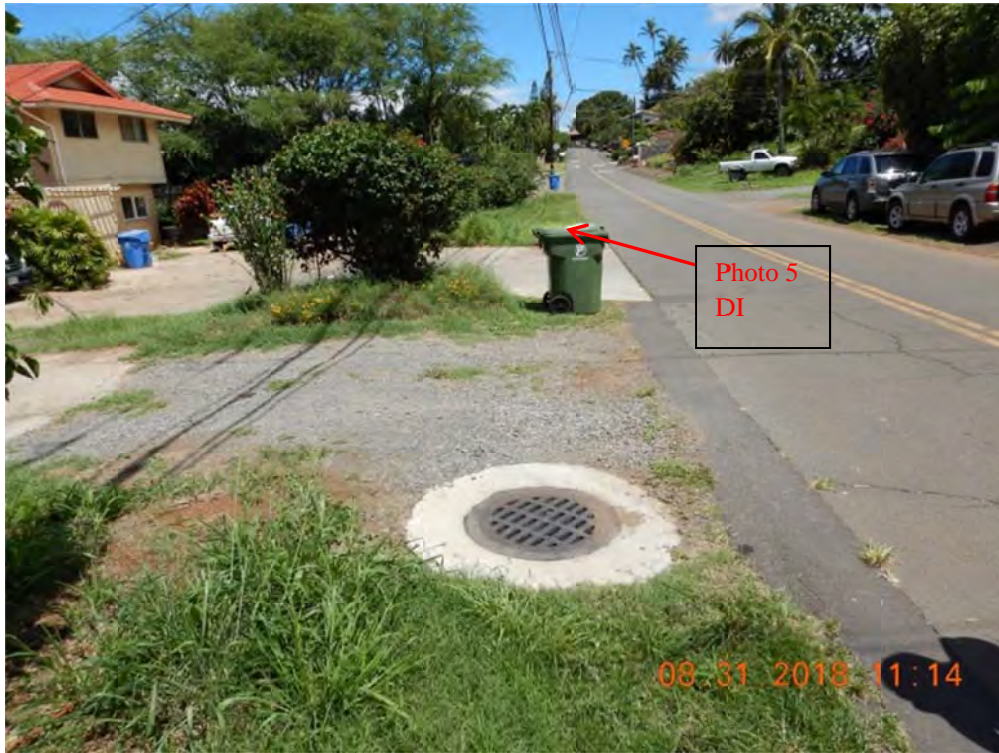
Photo 7: Another roadside drain inlet by private property TMK: 2-1-014: 087
