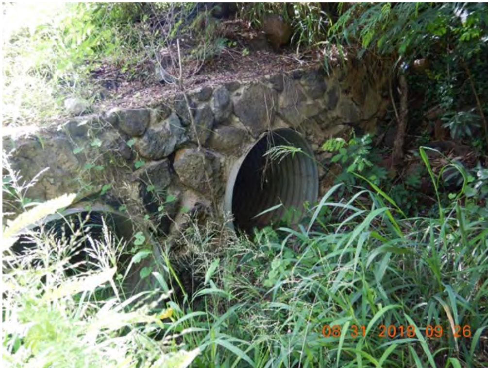
Photo 6: Stand on right bank, look toward Culvert 32 outlet
