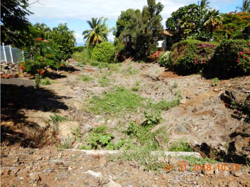
Photo 4: Stand on Mililani Pl, look toward downstream of Culvert 26
