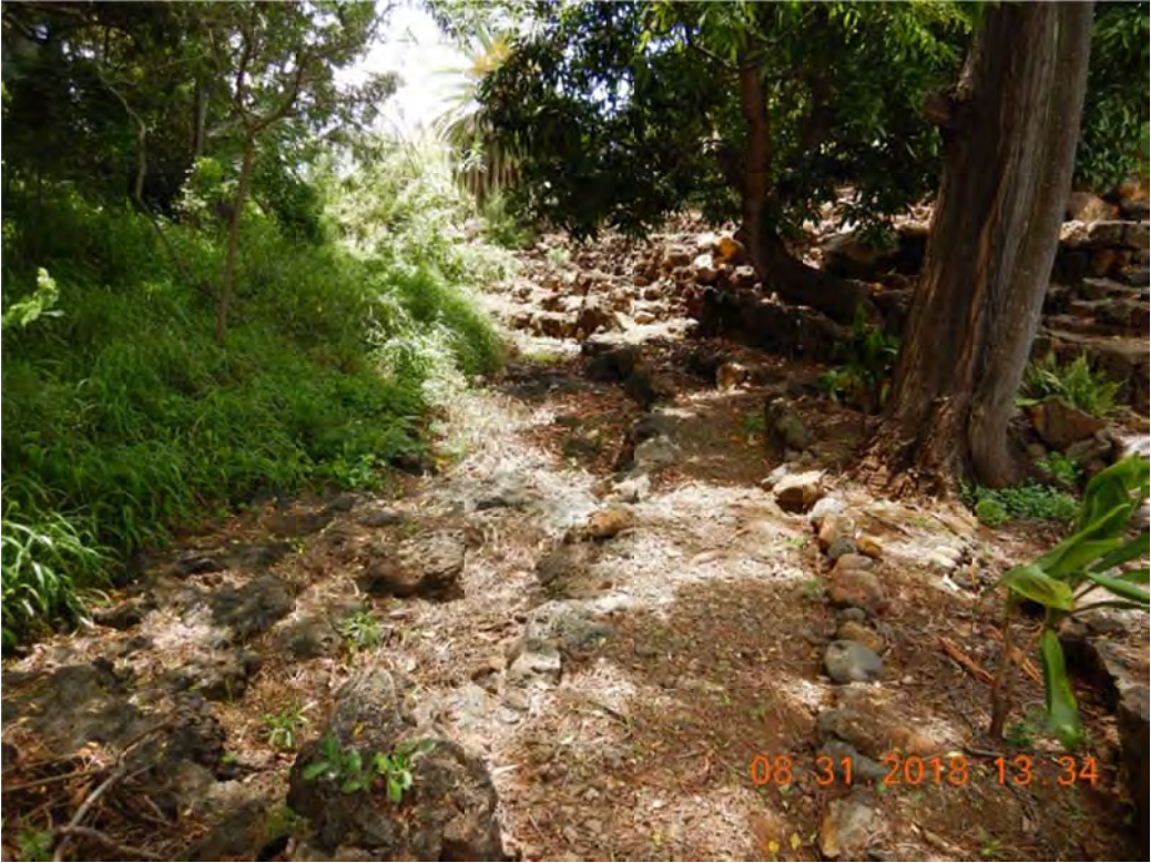
Photo 4: Look toward downstream of Culvert 7
