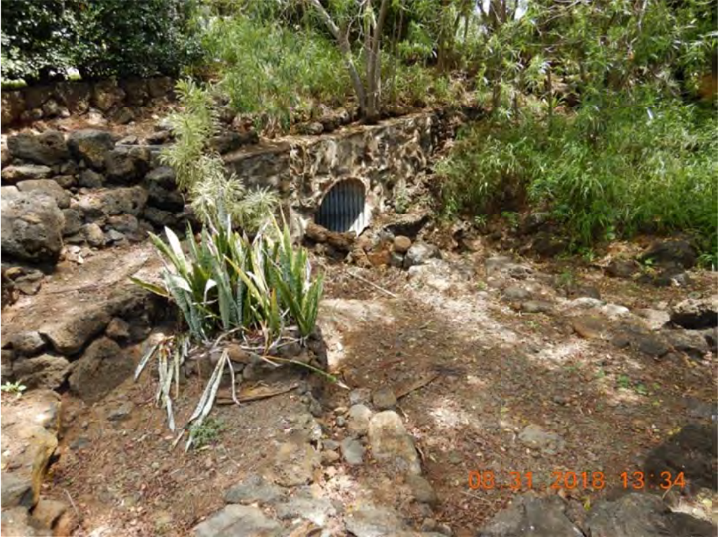
Photo 3: Stand on right bank, look toward Culvert 7 outlet
