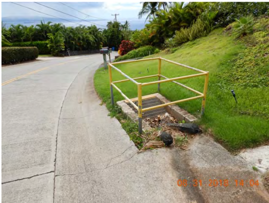
Photo 2: Close-up view of DI, filter sock was placed in front of DI
