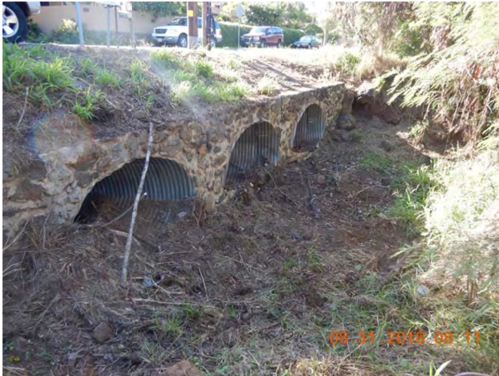
Photo 17: Stand on right bank, look toward Culvert 36 outlet
