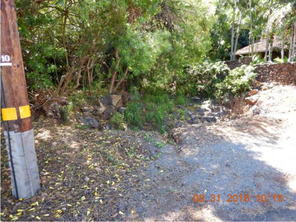
Photo 1: Stand on Mililani Pl, look toward upstream of Culvert 26
